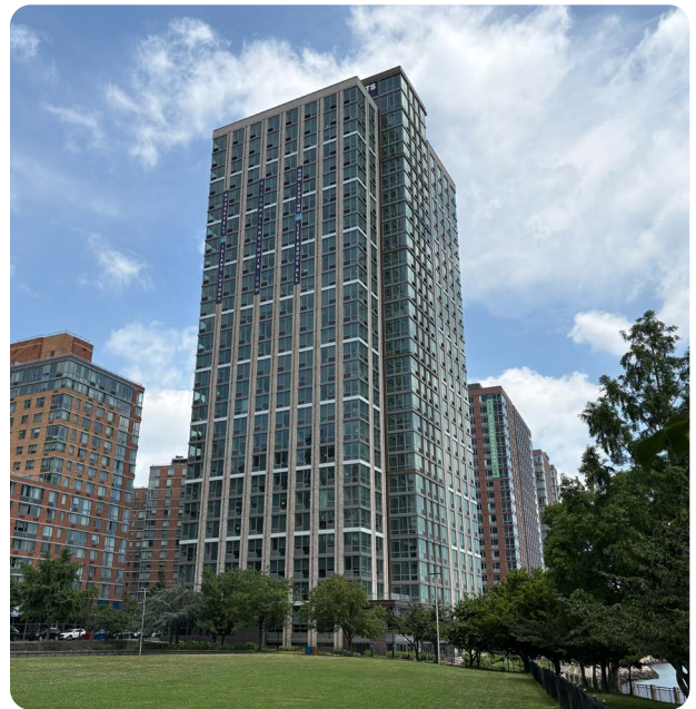
Building 9; 430 Main Street
